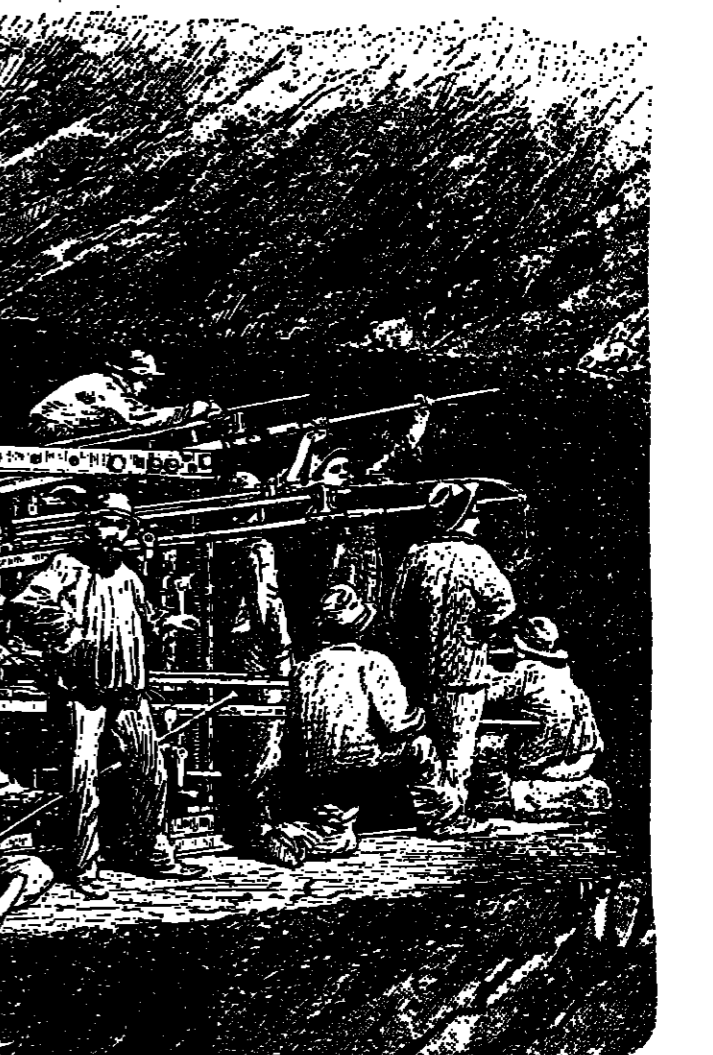
Sommelier's compressed air rock drilling machine revolutionised tunnelling techniques and made possible the 7.5 miles Mt. Cenis Tunnel, which was officially opened in 1871. It was the first to break through the Alpine barrier. No less indispensable was the financial vision of those who arranged the funding of this 14-year project, which cost £3 million.
